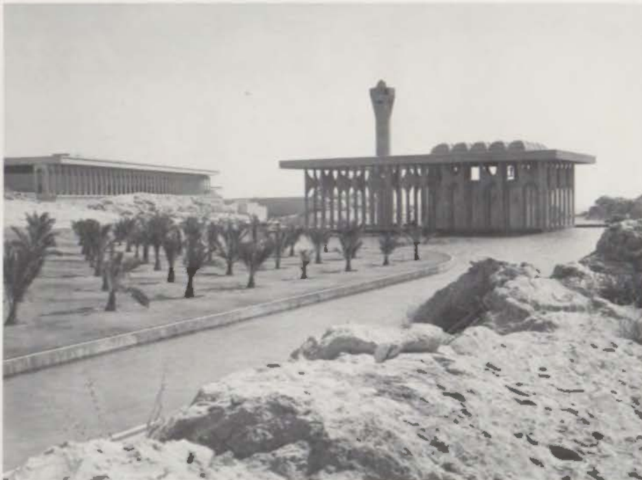
Mosque and minaret.
