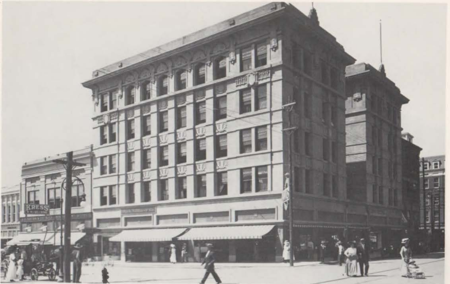
Roberts-Banner Building, Mesa and Mills Streets, completed about 1908, shown here about 1911. Constructed of reinforced concrete. Comprises five stories and two wings separated by a U-shaped light well.
