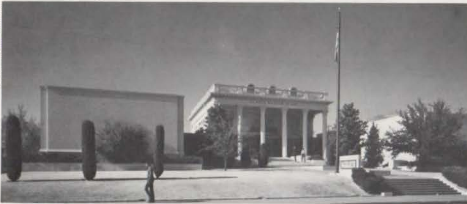
Turney residence with alterations and additions forming the El Paso Museum of Art (a project by the firm known at the time as Carroll & Daeuble & Associates).
