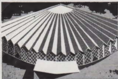
From the air, it's a lacy, shimmering fan. Congregation B'nai Israel Synagogue of St. Petersburg, Florida. Architect: Frank G. Bonsey, St. Petersburg. Structural Engineer: Joseph C. Rusello, Tampa, Florida. General Contractor: R. M. Thompson Company, Clearwater, Florida.
