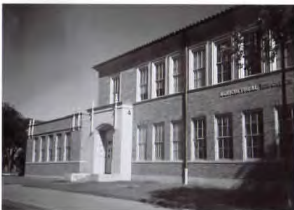
Bottom right: the Agricultural Engineering Building at Texas Tech
