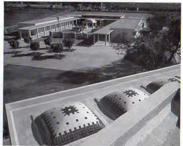
Above: tiled bovedas, seen from the roof of the theater, with the classroom wing in the distance
