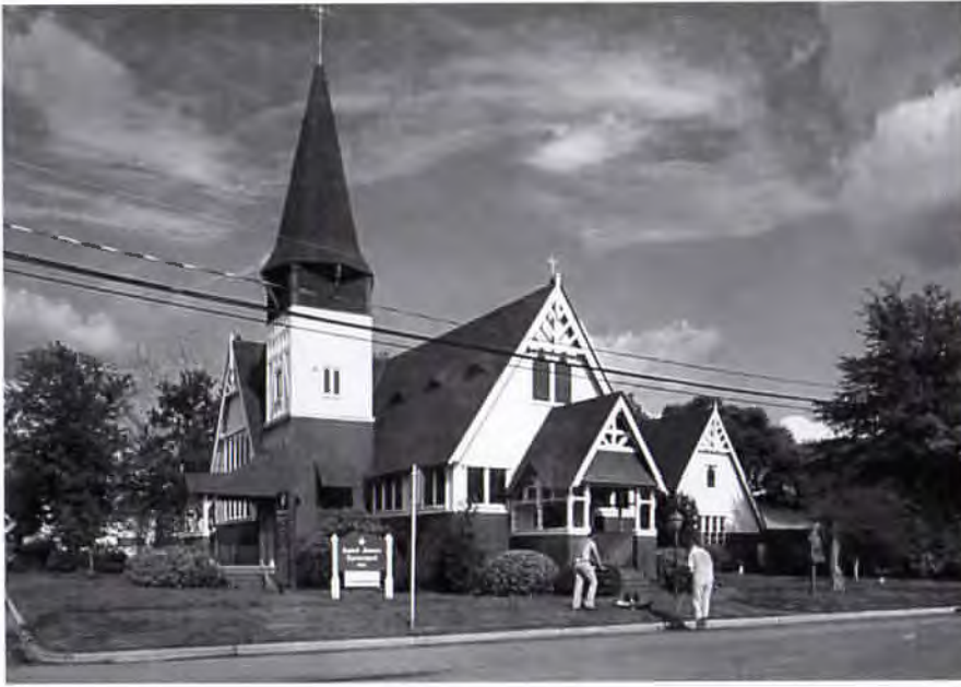
Above: Saint James Episcopal Church, LaGrange, 1885, Richard M. Upjohn; one of many styles imported from England, the Queen Anne made was characterized by medieval half-timbering, steep roofs, and elaborate carpentry. All-wood versions in the U.S. came to be known as the stick and shingle styles.
