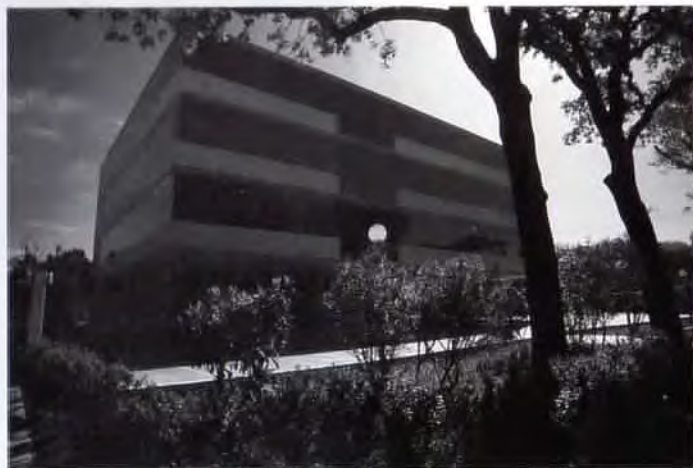
Careful siting eliminated unnecessary stairs and preserved a number of trees.
