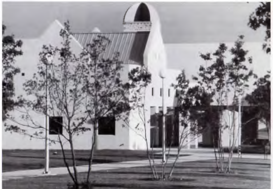
Palo Alto College, San Antonio, by JonesKell, Inc., and DeLara-Almond Architects, won an Honor Award.
