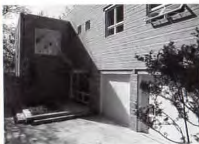
The jury liked the way McCall-Harris Architects made the entry to each unit private and distinct.
