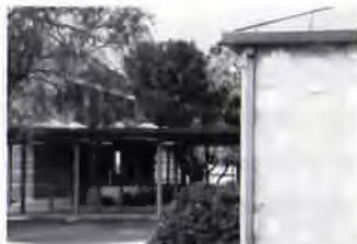
Welch Associates' additions, exterior
