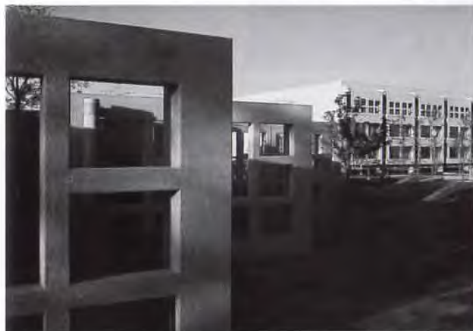
Precast sun screens provide a distinctive touch to an otherwise plain facade.
