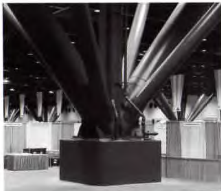
The center is built on 22 complex pipe columns.
