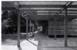
Pergola in church additions
