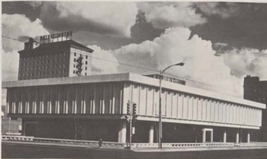
WEST TEXAS UTILITIES OFFICE BUILDING, SAN ANGELO LOVETT, SELLARS & ASSOCIATES, ARCHITECTS
