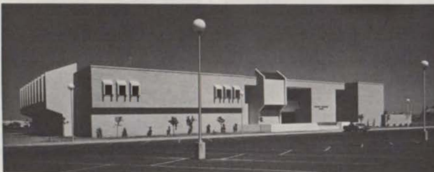
COMPOSITE TECHNOLOGY BLDG. ODESSA COLLEGE PETERS & FIELDS ARCHITECTS
