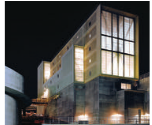
Ullrich Water Treatment Plant Extension
