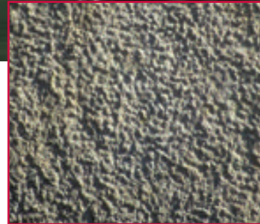
A brush-hammered finish created an aged texture.
