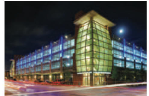
Austin Convention Center Parking Garage
