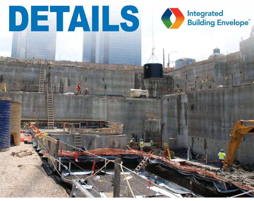
In building the Tarrant County College Trinity River East Campus in Fort Worth, Polyguard Underseal,<sup>®</sup> both Underslab and Blindside, was used as waterproofing. As you can see, lots of detailing was required. Detailed areas are where most leaks occur throughout the building envelope.
