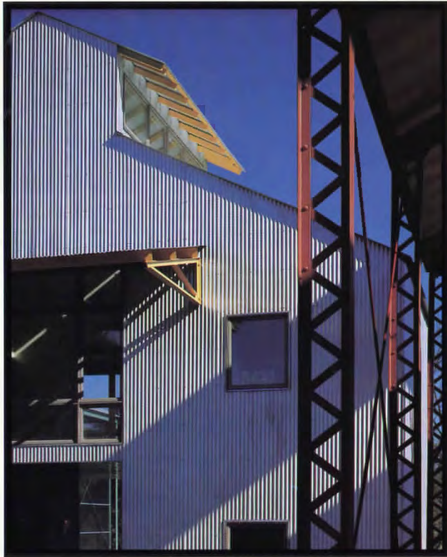
CARRARO HOUSE LAKE/FLATO ARCHITECTS
