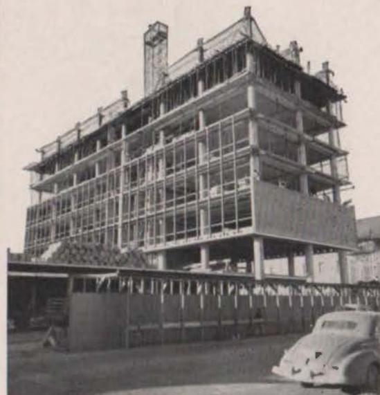
Upper photo shows 12-story section of Simms Building above the roof of block-square first floor. The floors throughout are 6-in. thick reinforced concrete using a wide beam design and cantilevered 5 ft. outside the supporting columns. Architects and engineers: Flatow-Jason Moore. Contractor: Lembke, Clough & King, Inc. Both of Albuquerque.
