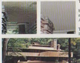
Thoro System Products be used throughout. After sandblasting, contractors Mariani and Richards brought the surface back to its original form with Thorite, a non-slumping, quick-setting patching material (mixed with Acryl 60 for enhanced bonding and curing).
