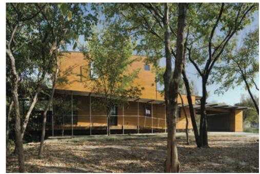
On the west – or "dry" – side of Urban Reserve, Dan Shipley, FAIA, designed a house that floats above the ground on 60-foot-long steel beams. The photo shows the south facade of the house.
