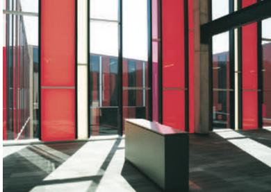
also used on the perimeter of the village and the red-tinted glass used only on the courtyard side. The three types of opaque glass — white and two shades of red—resemble the narrow color range of a geode. Furnishings in the common areas repeat the red hues of the fenestration.
