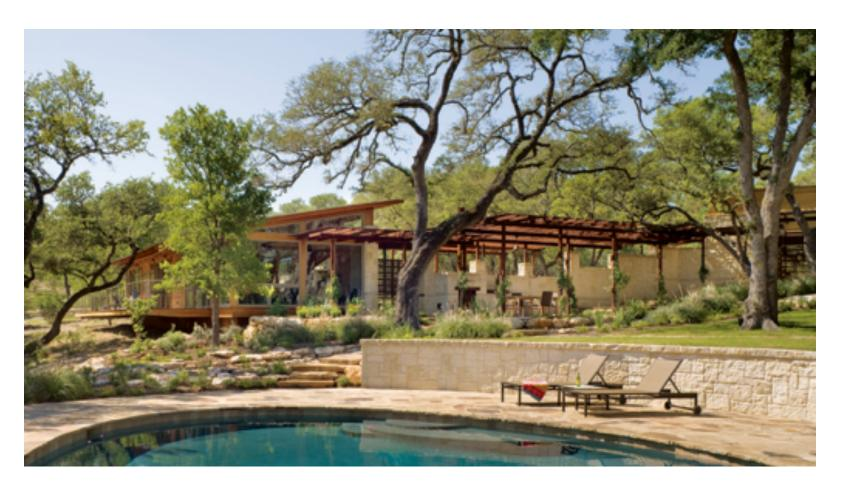
(preceding spread, left and right) Shaded by weathering steel pergola, an exterior walkway connects the family residence with the guest quarters. Deep overhangs shield the glazing along the southwestern elevation of the main house.
