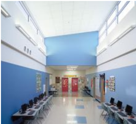
(top left and right) The hard edges of the building envelope give way inside to colorful interior finishes and playful forms animated by abundant natural light. (above) Clerestories set high along the wide corridors help create optimal conditions for additional learning areas.
