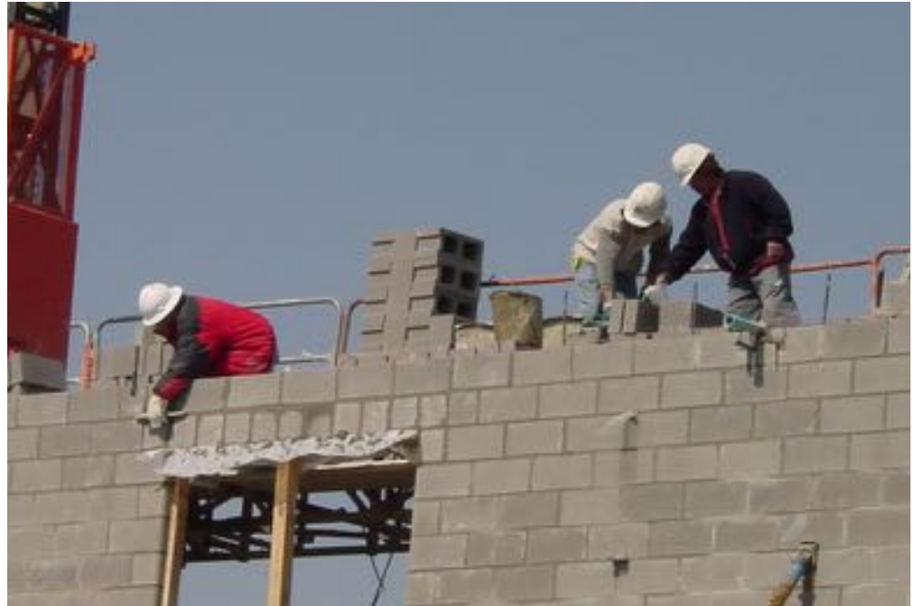
The biggest potential advantage of masonry bearing-wall buildings is their efficiency. The masonry works simultaneously as architectural element, building envelope, and structure.
