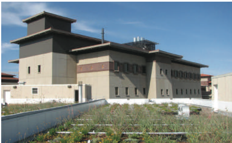
The Biology Building was retrofitted last year with a modular green roof system of pre-planted trays and monitoring equipment to gather data on the building's energy performance. UTEP's director of campus planning and construction championed the project to convince wider application of green roofs across the Southwest.
