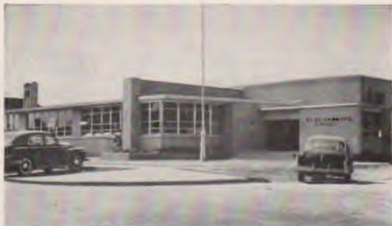
Stran-Steel Framing was used in walls, roof and partitions in the St. Elizabeth School, Alice, Texas. Wade, Gibson & Martin, architects.
