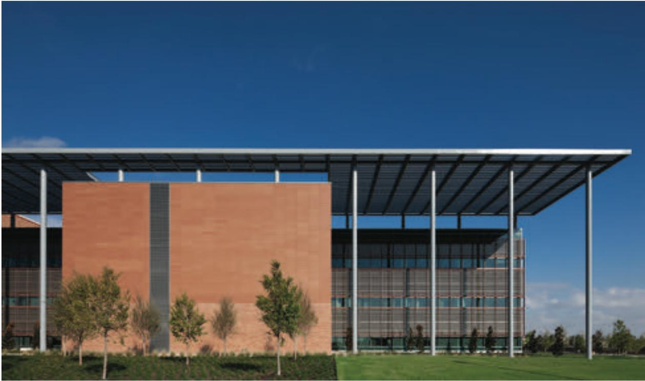
**Clockwise from top** A large canopy is supported by steel columns that taper slightly over their length. In addition to providing shade, this canopy helps tie together the various masses of the expansion. In addition to providing natural light, floor-to-ceiling glass helps connect patient rooms to the outside world. Generous interior “malls” help orient visitors and patients within the 750,000-sf facility.
