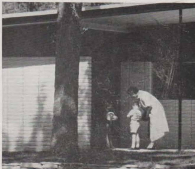
Design interest is achieved with coarse-textured block laid in a stacked bond
